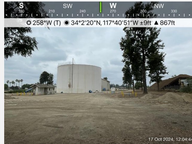
Photo 2. Overview of site, taken from northeastern corner.
