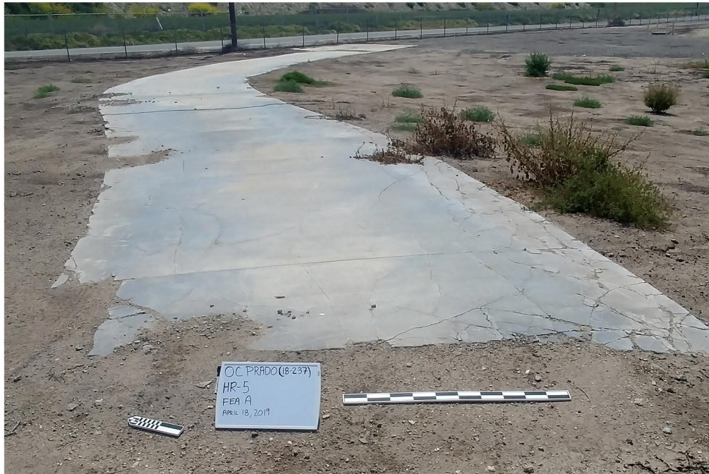
Plate 5.2.4-2: Overview of the Feature A concrete driveway at Site CA-SBR-33,116H, facing southeast.
