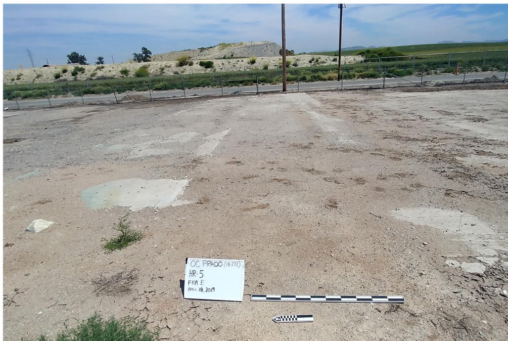
Plate 5.2.4-6: Overview of the Feature E concrete driveway at Site CA-SBR-33,116H, facing east.
