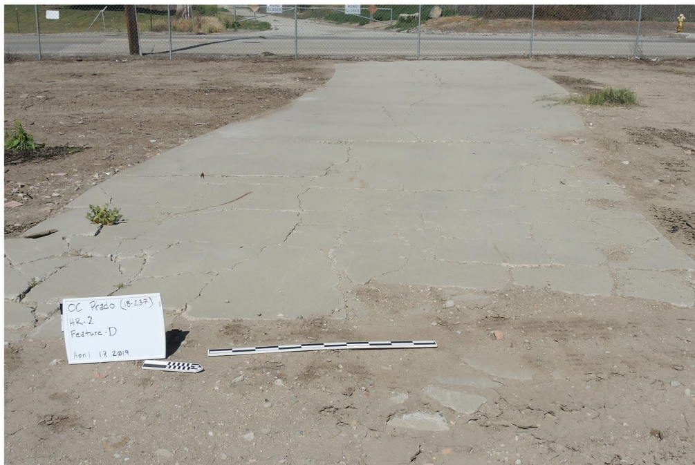
Plate 5.2.1-18: Overview of the Feature D concrete driveway at Site CA-SBR-33,113H, facing west.
