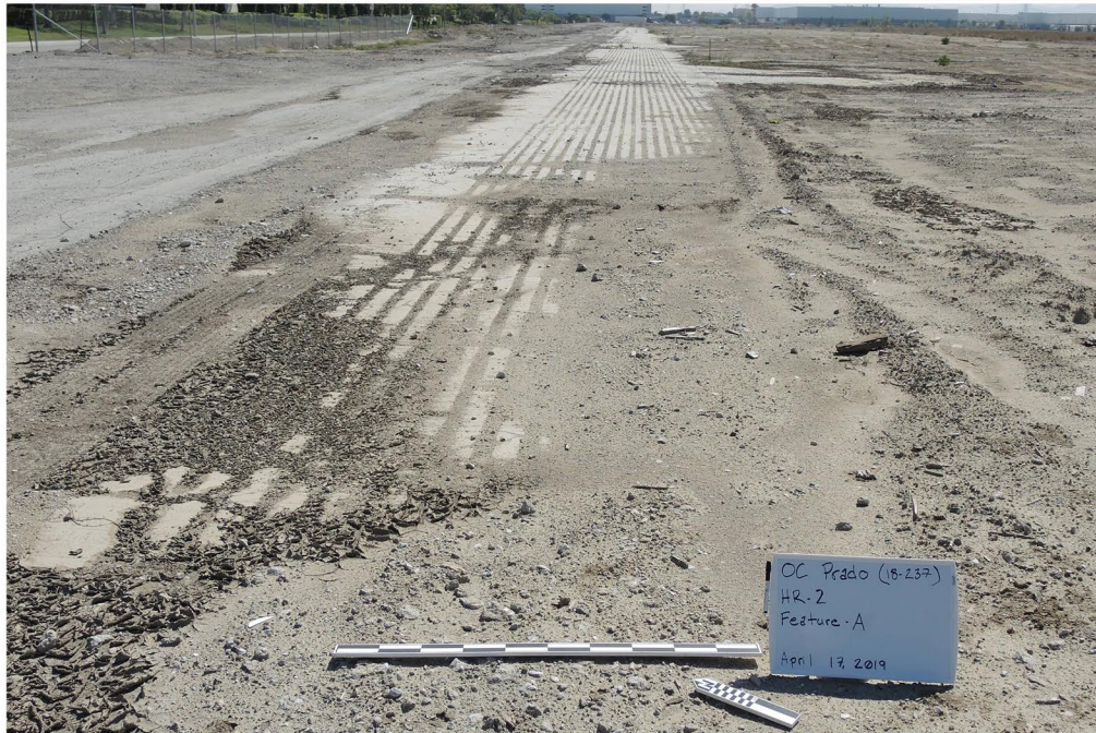
Plate 5.2.1-15: Overview of Feature A feed alley foundation remnants at Site CA-SBR-33,113H, facing northeast.
