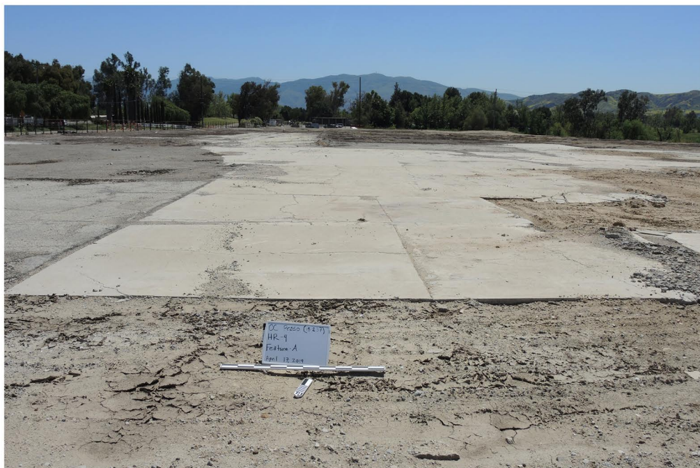
Plate 5.2.2-20: Overview of Feature A slaughterhouse facility foundation remnants at Site CA-SBR-33,115H, facing south.
