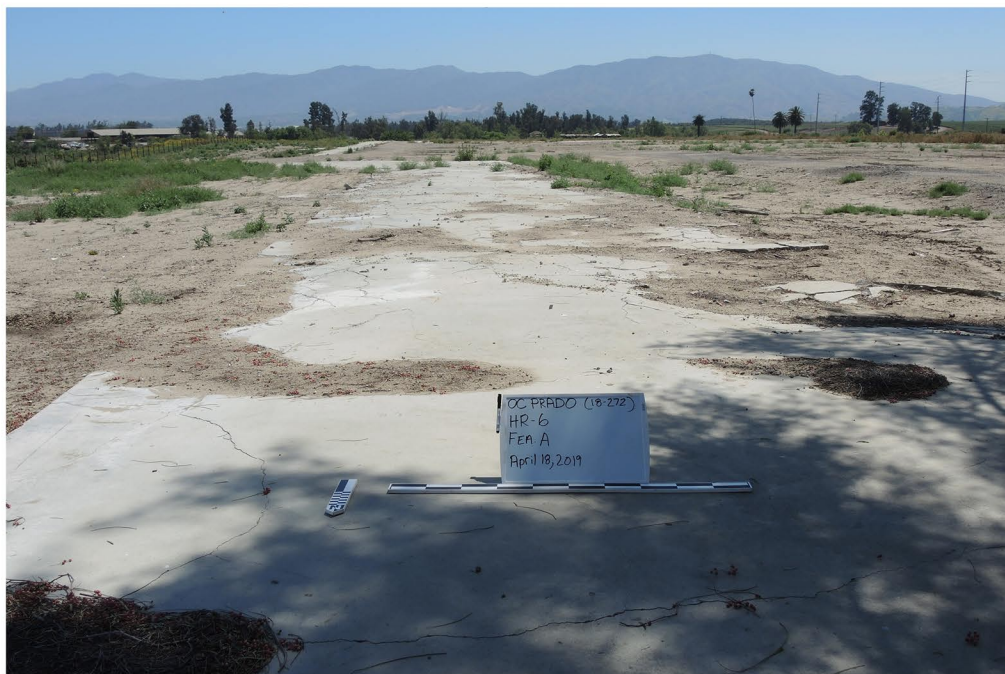
Plate 5.2.5-1: Overview of the Feature A concrete driveway at Site CA-SBR-33,117H, facing south.
