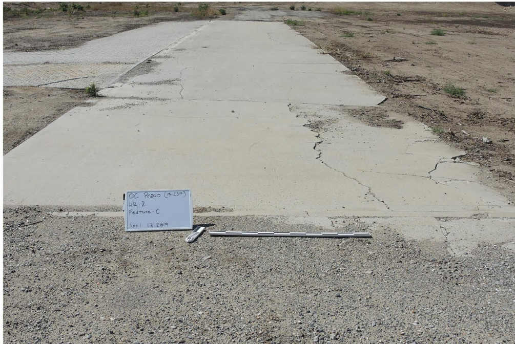
Plate 5.2.1-17: Overview of Feature C feed alley foundation remnants at Site CA-SBR-33,113H, facing south.
