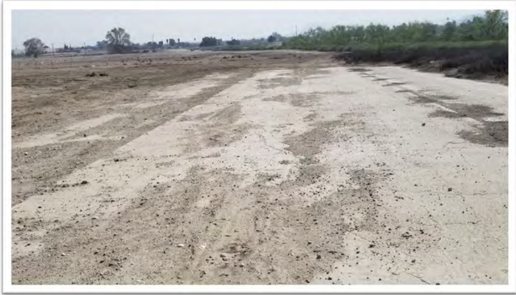
Photo 17. Concrete Pavement Related to Former Dairy Operations on the Property.
