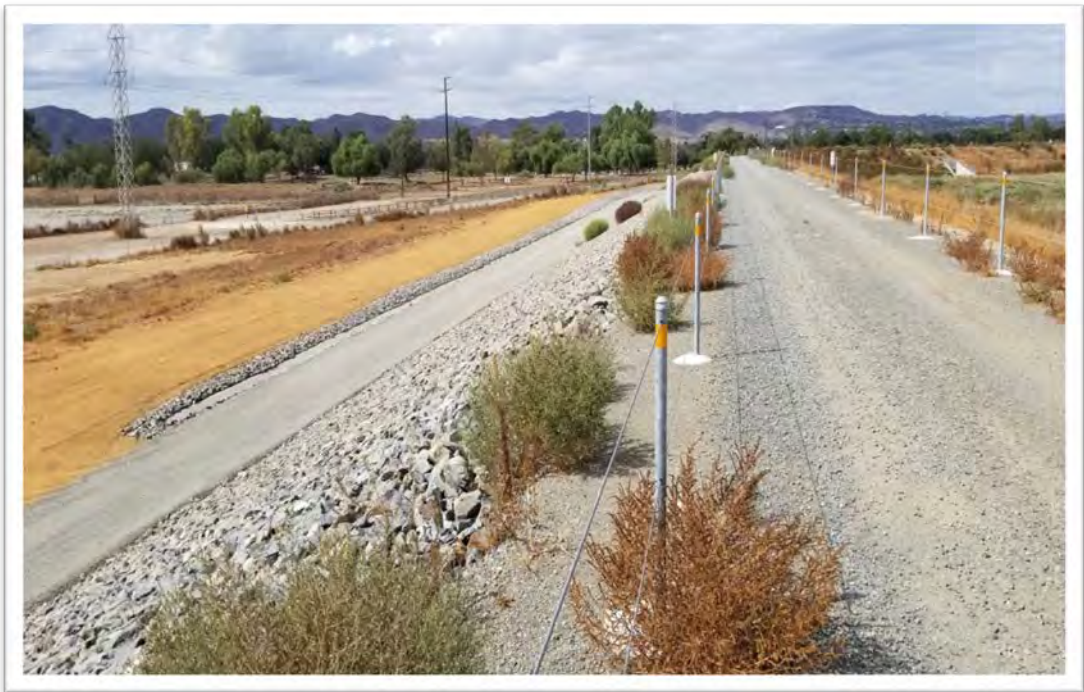
Photo 12. View From North/South Access Showing Adjacent Paved Road.
