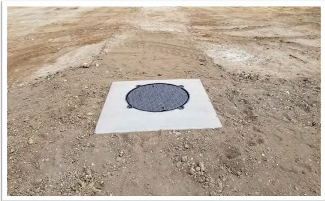
Photo 4. Apparent Storm Drain Manhole Access on the Site.
