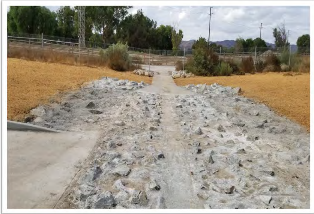
Photo 9. Concrete/Rock Apron for Flood Control Outlet to Cucamonga Avenue.
