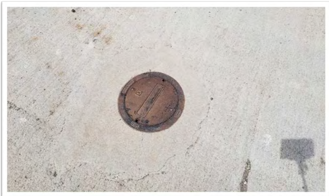
Photo 10. Unlabeled Metal Access Plate in Paved Area on the Site.
