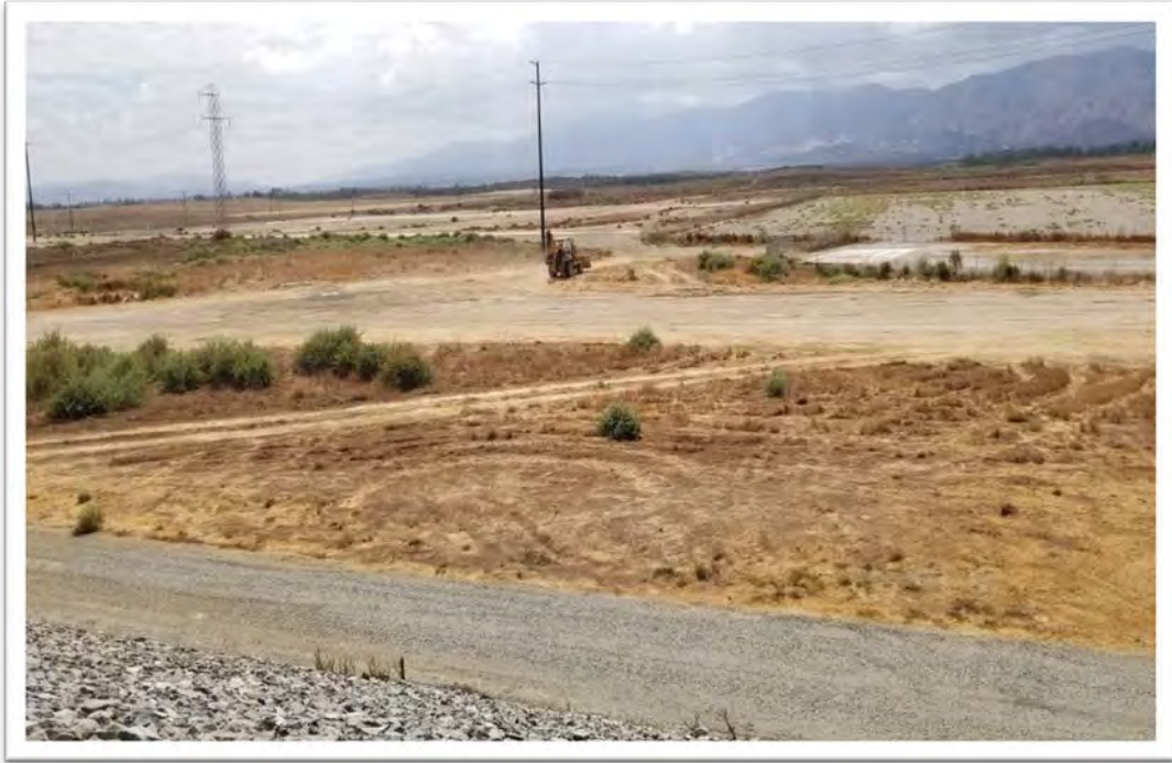
Photo 19. View of Site Showing Adjacent Undeveloped Area.
