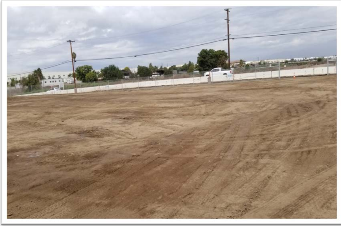
Photo 9. Northwest Portion of the Site Looking Towards Pine Avenue.
