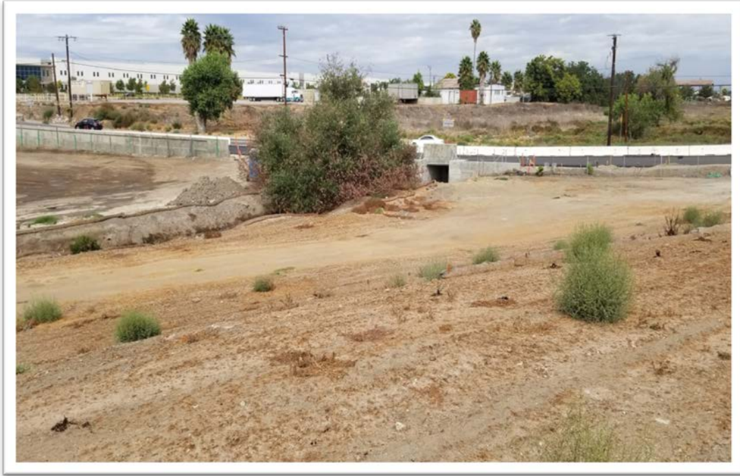
Photo 19. View of Drainage Channel Along the Western Portion of the Site.
