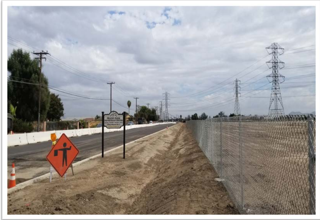
Photo 5. View East on Pine Avenue from Intersection of Pine/Johnson Avenues.
