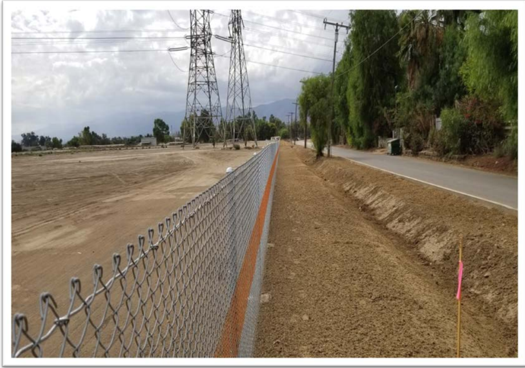
Photo 3. View South on Johnson Avenue Showing Graded Drainage Channel.
