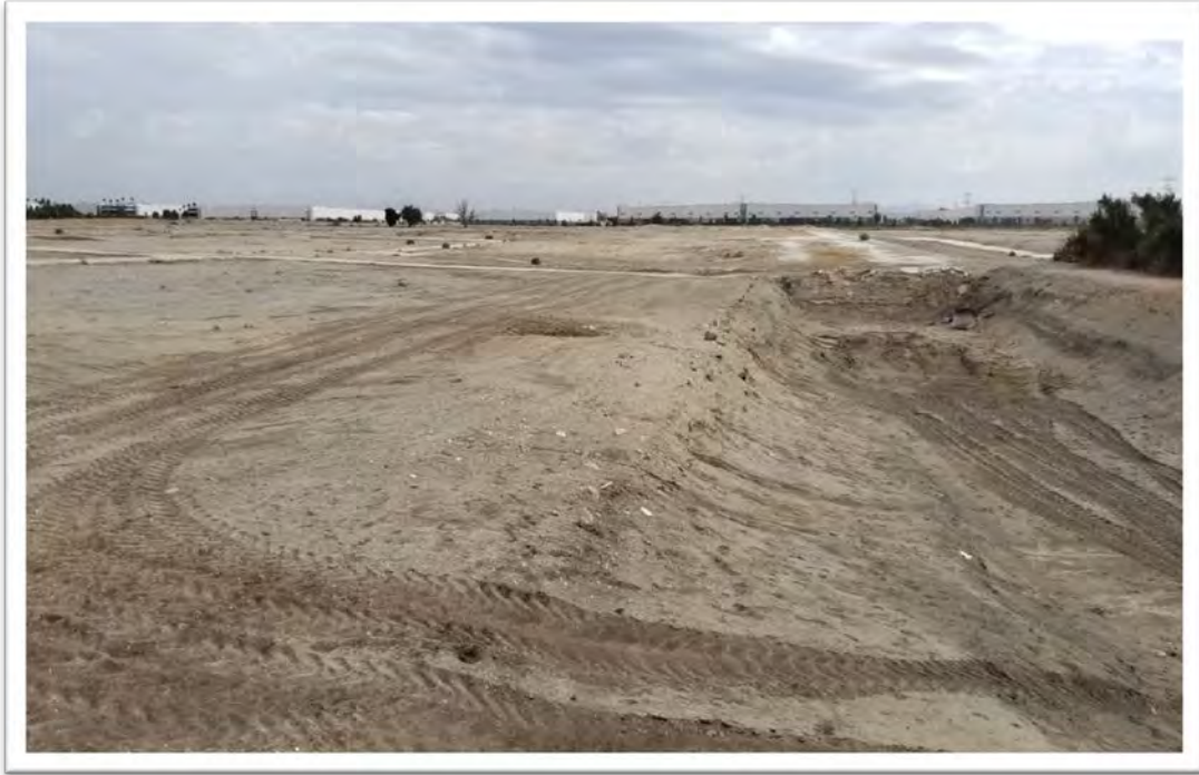
Photo 11. View East Across 95 Acre Parcel.
