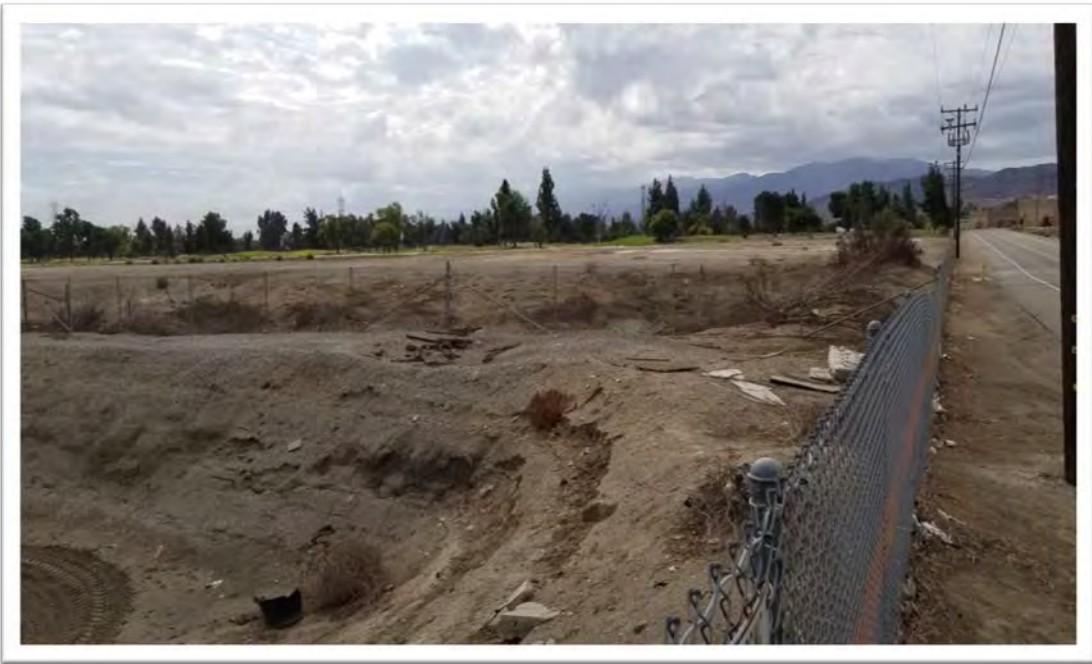
Photo 8. Impoundment Area in Southwest Portion of the Site.
