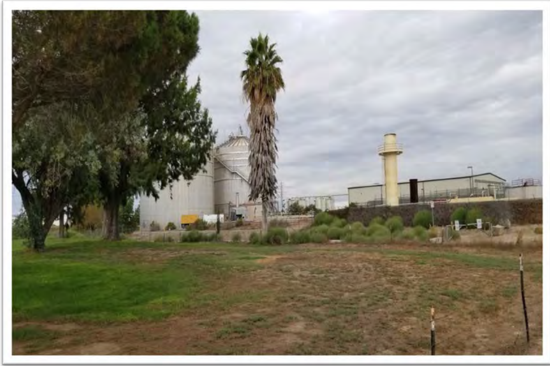
Photo 5. Commercial Facility Located at the NWC of Flower Street and Mountain Avenue.
