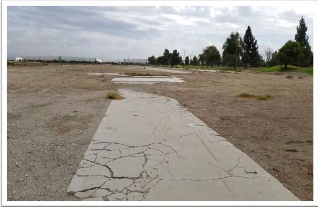
Photo 13. View of Central-West Portion of the Site Showing Concrete Pads.
