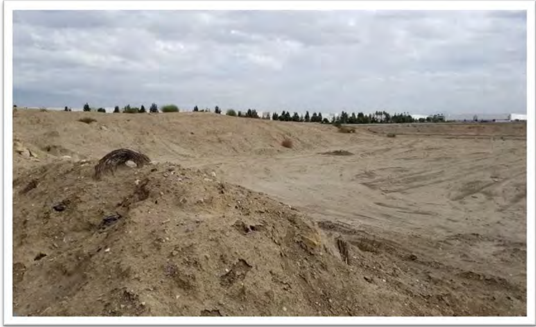
Photo 6. Bermed Soil Area on the 95 Acre Parcel.
