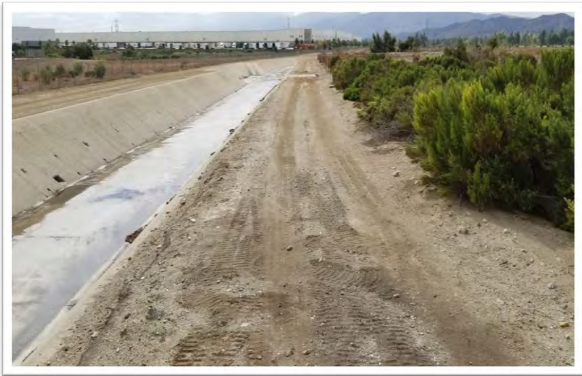
Photo 20 Concrete Channel and Warehouse Buildings in Eastern Portion of the Site.
