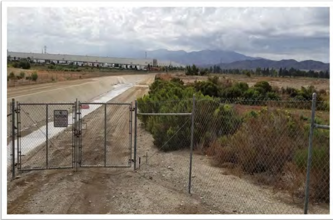
Photo 16. Concrete-Lined Drainage Channel Along Eastern Boundary of the Property.
