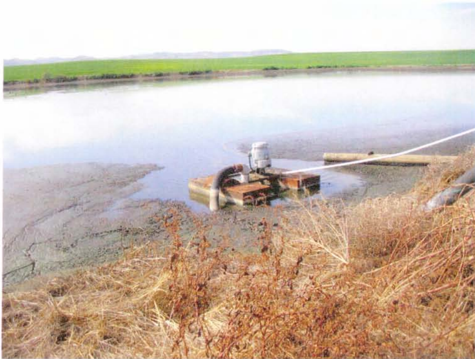
Overview of Holding Pond A.
