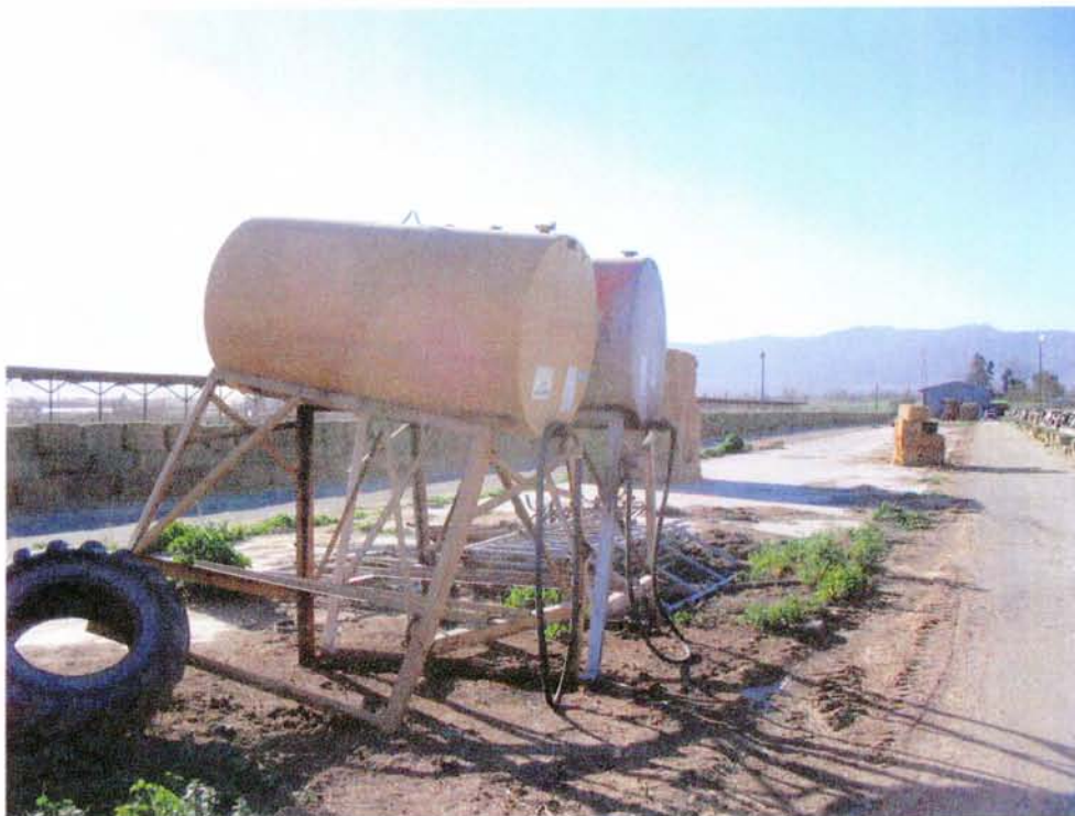
500-gallon diesel fuel ASTs by the animal pens near dairy.
