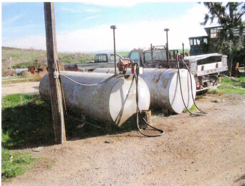
1,000-gallon AST's of unleaded gasoline and diesel fuel at barn.
