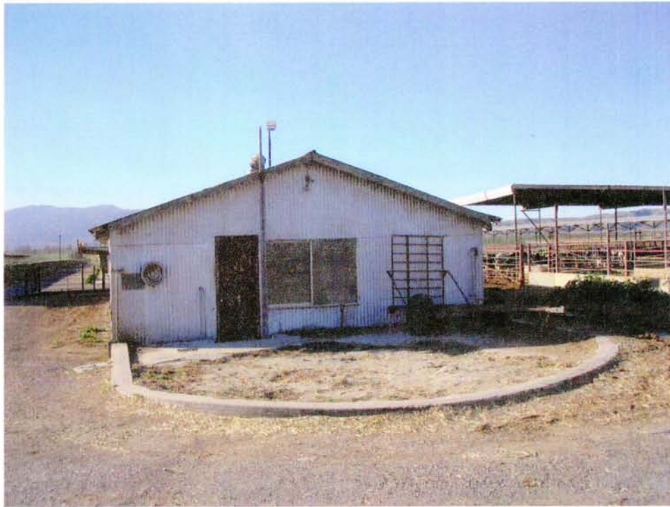
Overview of former UST area.
