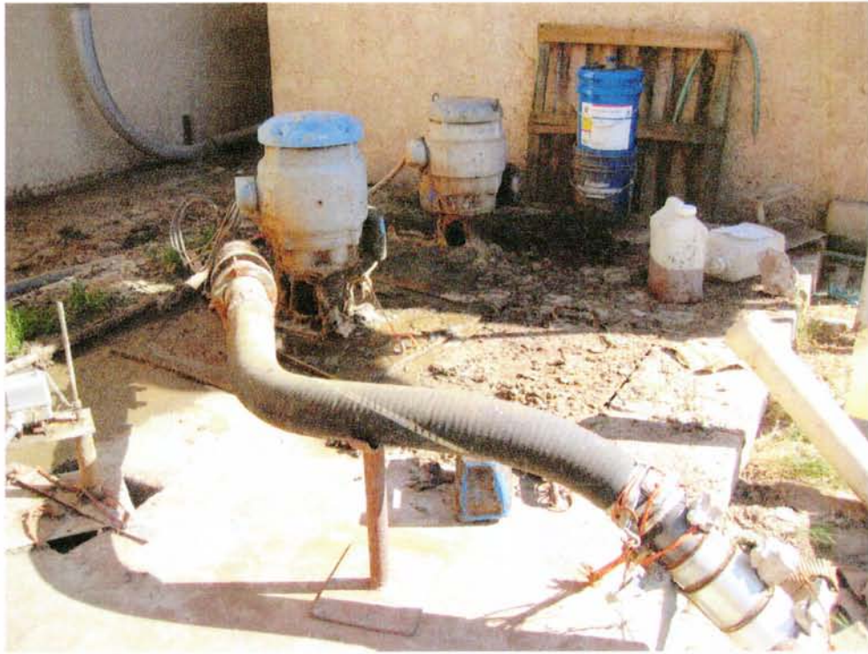
Overview of sump adjacent to milking barn.
