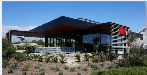
Local business with on-site dining
