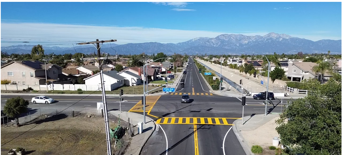
Chino Ave at Cypress Ave, looking north
