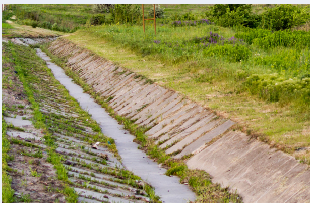
Flood Control Channels
