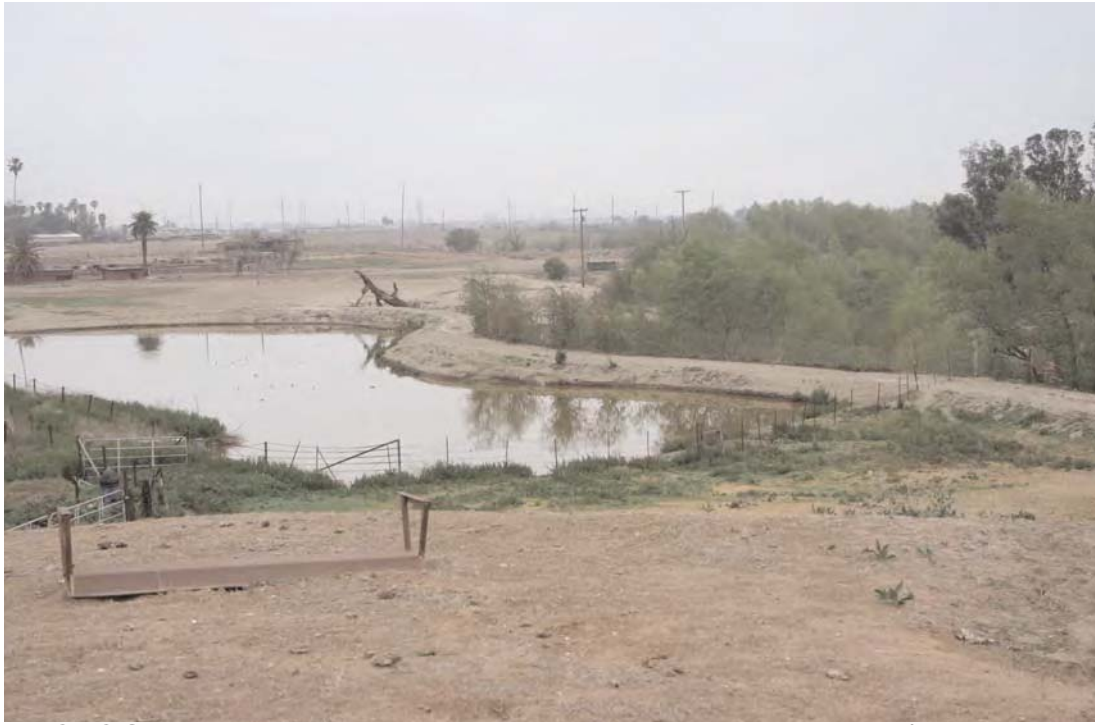
PHOTOGRAPH 3: Agricultural pond created by excavating and/or diking dry land. Note prominent berm that separates agricultural pond from Mill Creek and maintains hydrologic separation. Pond is maintained and generally supports little or no vegetation as shown.
