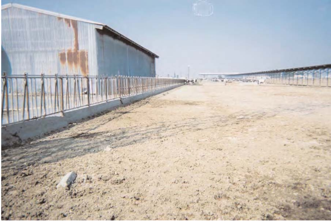
PHOTOGRAPH 3. North-facing view of abandoned dairy facilities near the northern edge of the project site.
