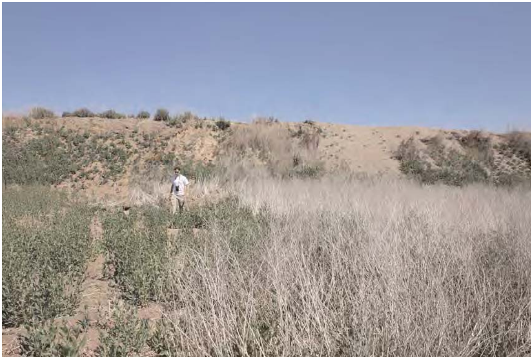
PHOTOGRAPH 6: View of berm constructed to create pond shown in above photo. Note lack of outlet that would allow water to reach Mill or Chino Creeks.
