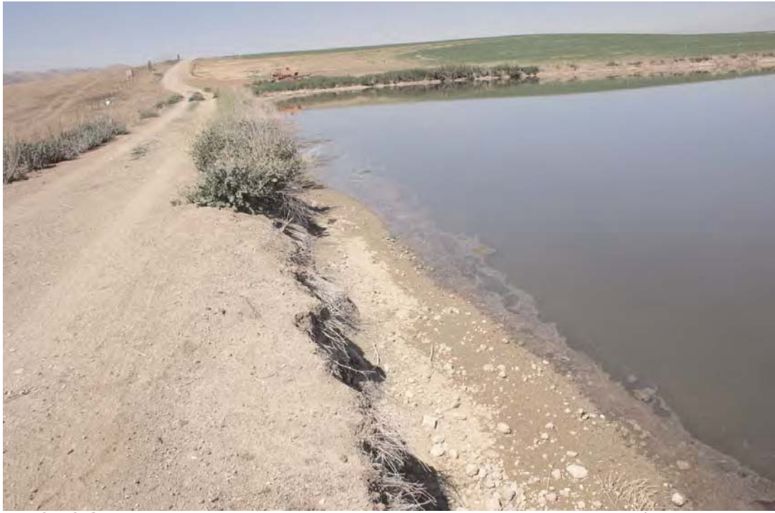
PHOTOGRAPH 5: Agricultural pond created by excavating and/or diking dry land. Note prominent berm that separates agricultural pond from Mill or Chino Creek and maintains hydrologic separation. Pond is maintained and generally supports little or no vegetation as shown.
