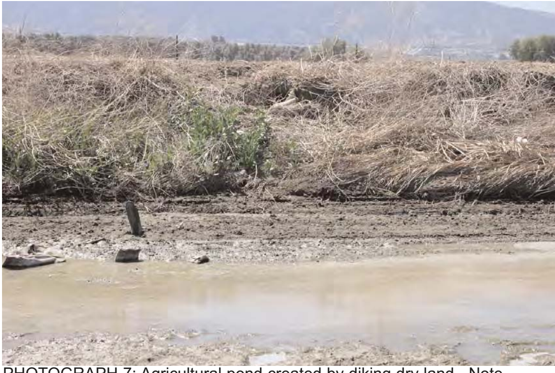
PHOTOGRAPH 7: Agricultural pond created by diking dry land. Note prominent berm that separates agricultural pond from Chino Creek and maintains hydrologic separation. Pond is maintained and generally supports little or no vegetation as shown. Outlet pipe to berm can be seen near top of berm (next to plastic).
