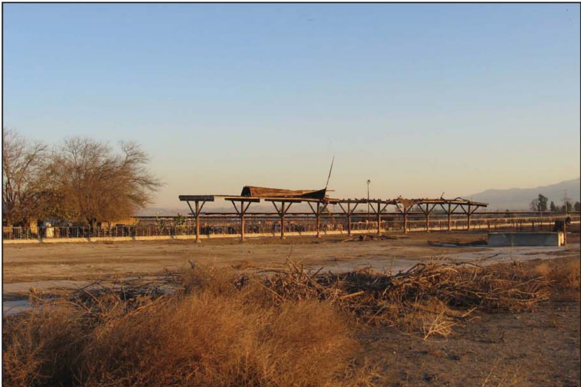
Photograph 22: Southeastern view of the Project site and active dairy operations.
