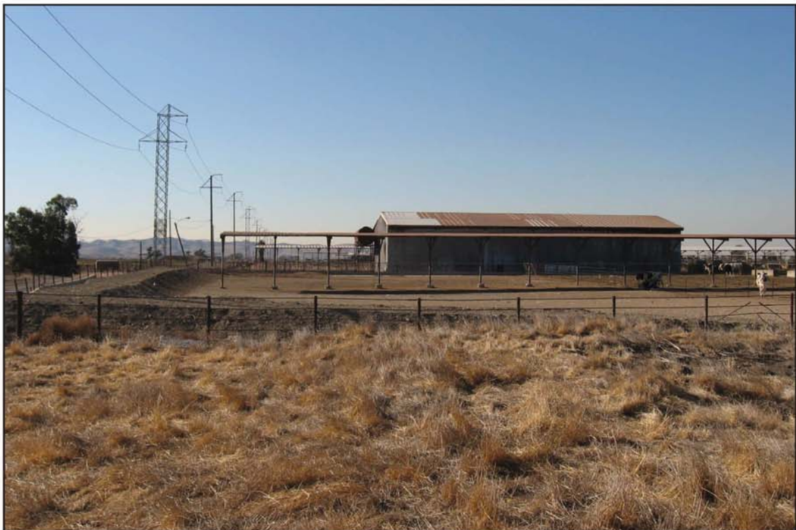
Photograph 2: Western view of the Project site showing the active dairy operations and transmission lines running east-west within and along the boundary of the Project site.
