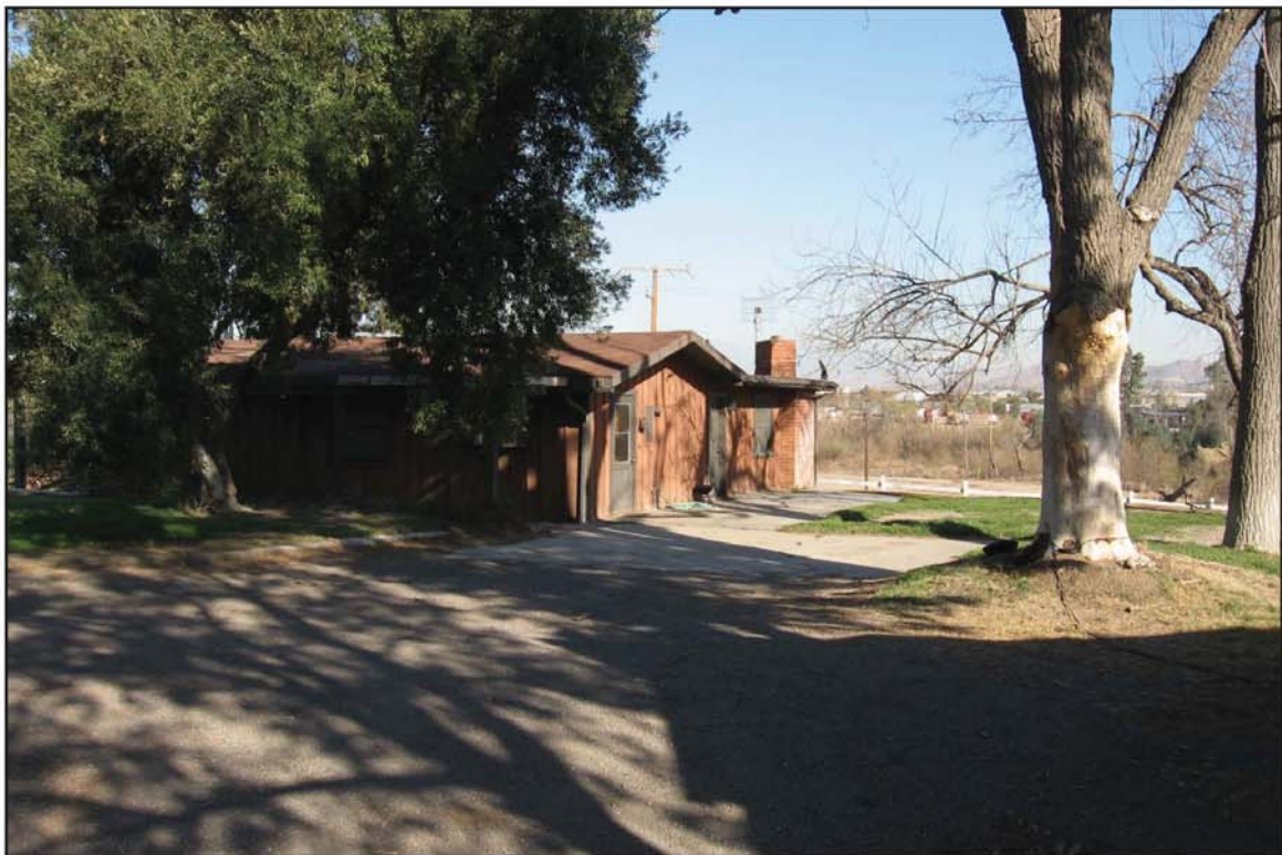
Photograph 6: Northeastern view of the ranch house located on a knoll in the eastern-central portion of the Project site.
