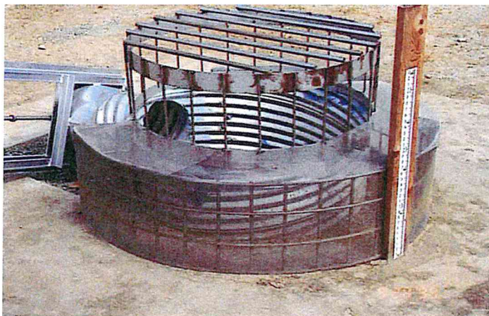
Figure 1 Example of Extended Detention Outlet Structure
