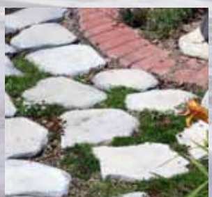
Permeable pavement allows water runoff to infiltrate through the soil and prevents most pollutants from reaching the storm drain system.
