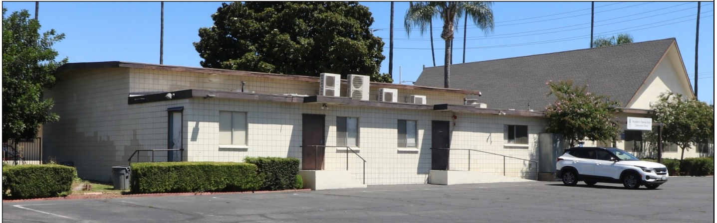
Rear addition, view northeast (9/13/24).
