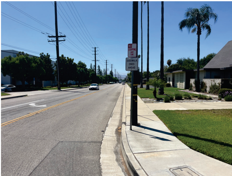
Photo 4: Eastern Project Site Boundary along Oaks Avenue, Facing South
