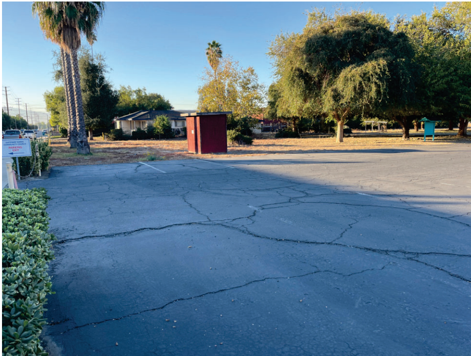
Photo 6: Developed Portion of the Project Site, Facing Southwest
