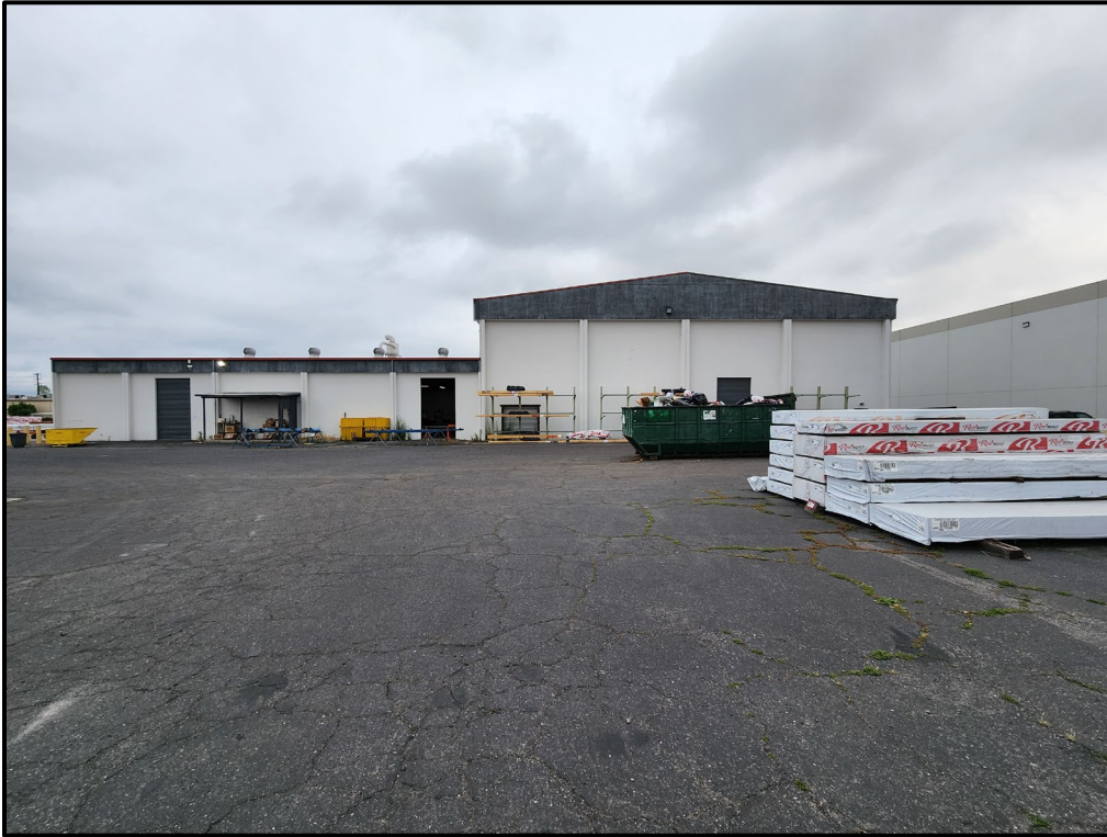
Plate 3.3–10: East façade of Building 3, facing west.
