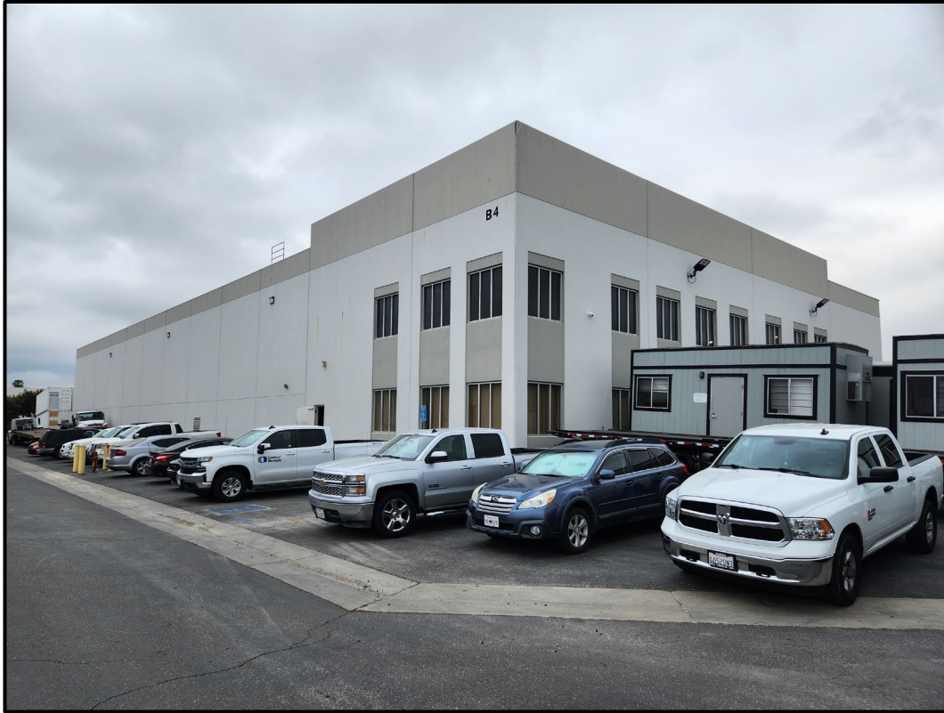
Plate 3.2–3: Overview of the existing 2006 United Rentals building within the northern half of the project, facing northwest.
