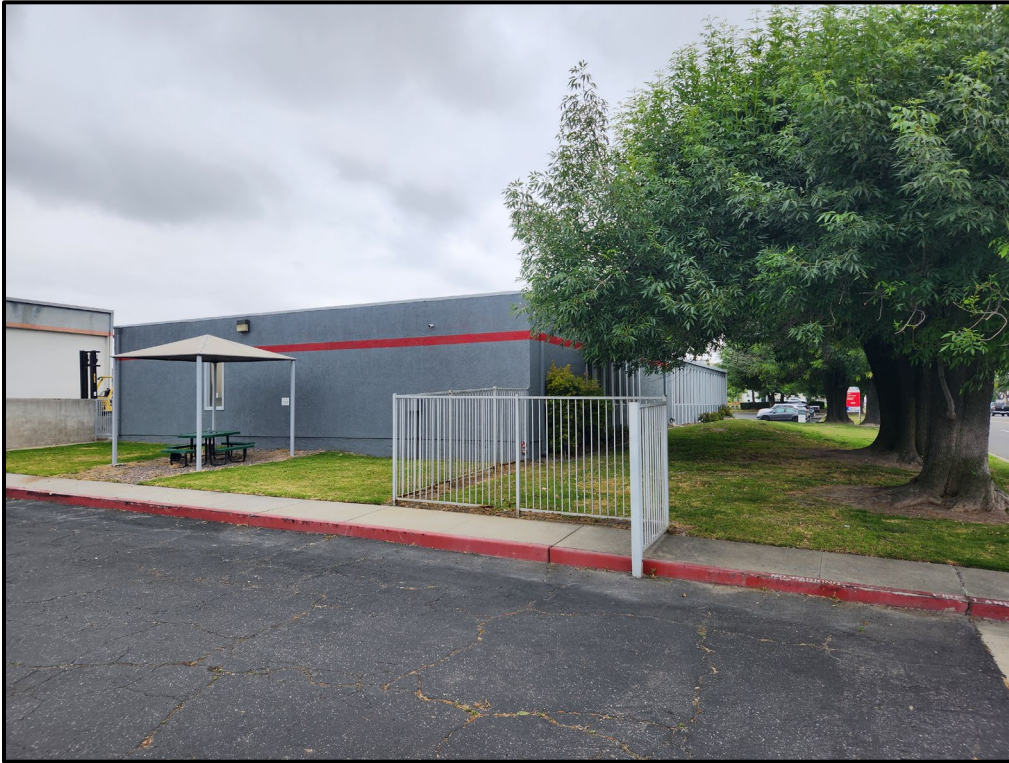
Plate 3.3–3: West façade of Building 1, facing northeast.
