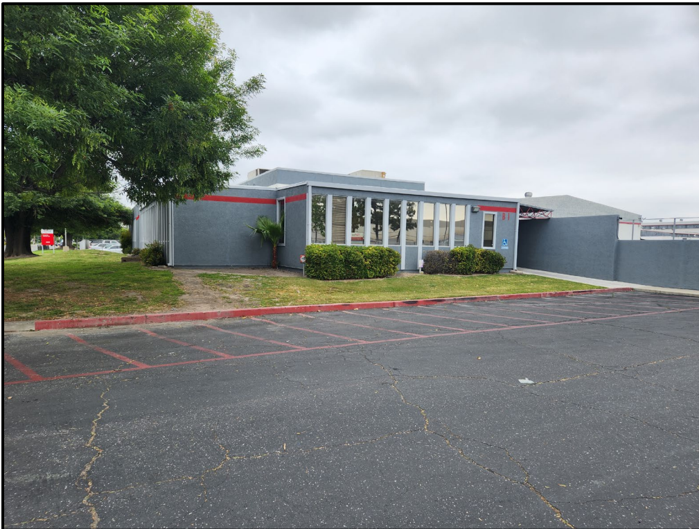
Plate 3.3-2: East façade of Building 1, facing northwest.
