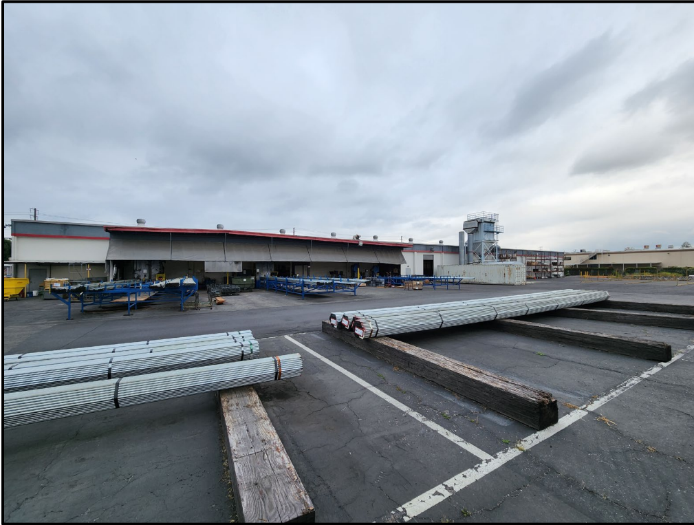
Plate 3.3–6: North façade of Building 2, facing southwest.
