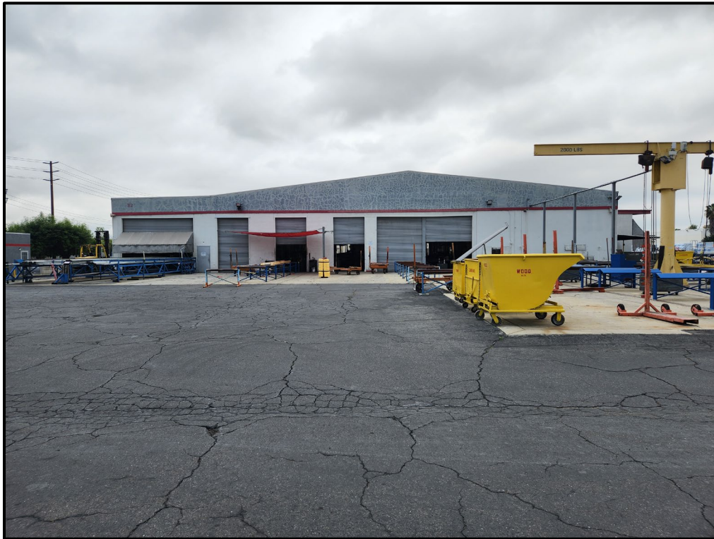
Plate 3.3–5: East façade of Building 2, facing west.
