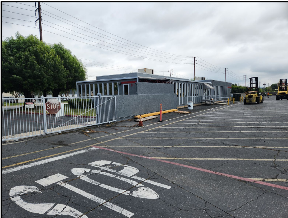
Plate 3.3–4: North façade of Building 1, facing southwest.
