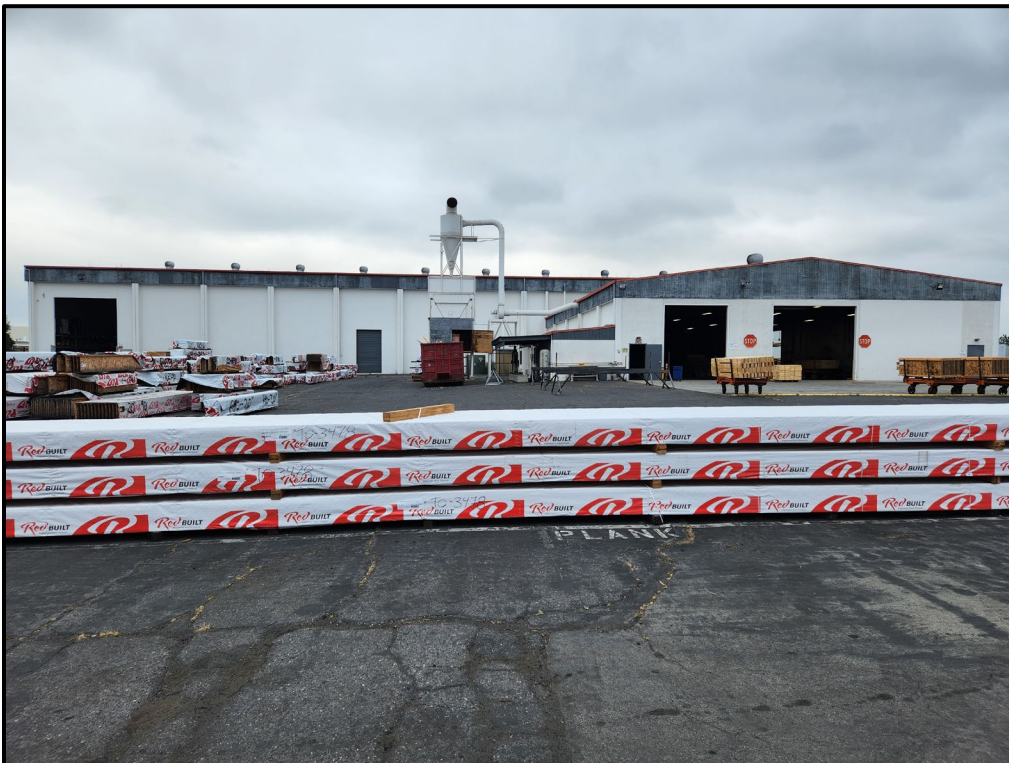
Plate 3.3-9: South façade of Building 3, facing north.
