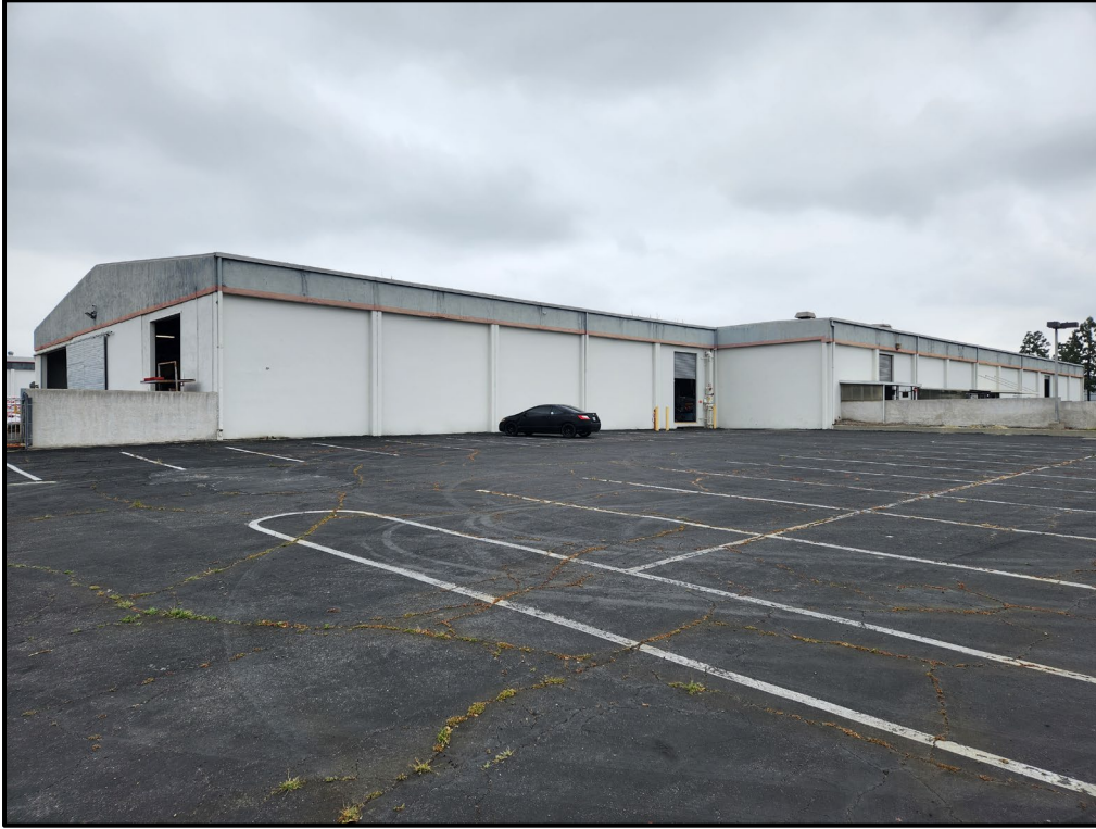
Plate 3.3-8: South façade of Building 2, facing northeast.
