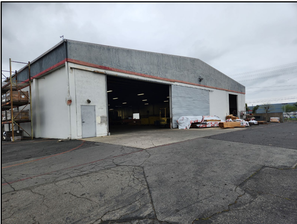
Plate 3.3–7: West façade of Building 2, facing southeast.
