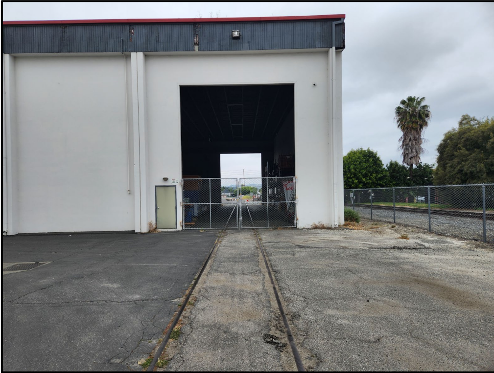
Plate 3.3–12: Railroad siding extending through Building 3, facing south.
