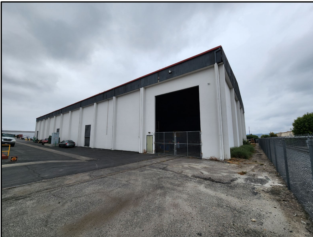
Plate 3.3–11: North façade of Building 3, facing southeast.
