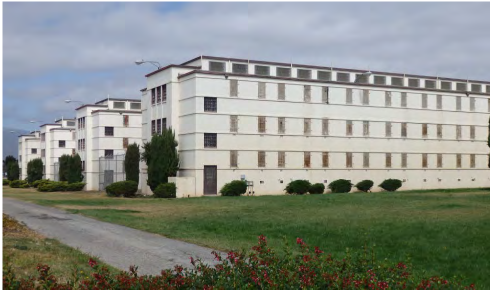
Exhibit 2. CTF-Central. Designed 1949, opened 1951.
