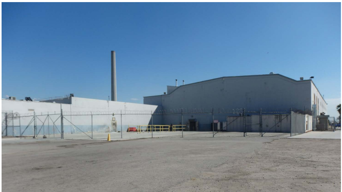
Rear of culinary building. Bakery addition to shorter northern building at far left.
