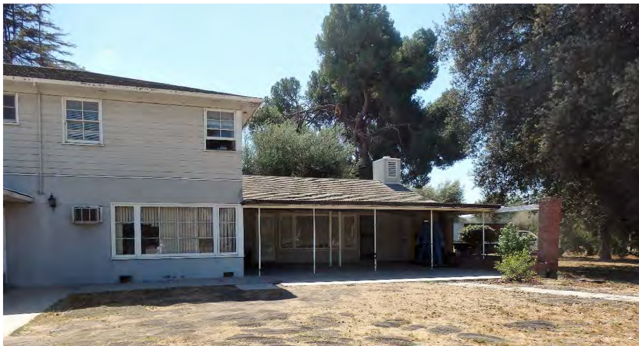
Rear of house, looking southwest at covered porch.
