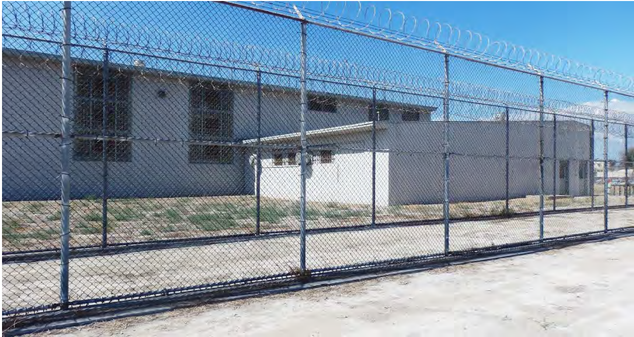
Unit 5 and Birch Hall, constructed early 1960s.
