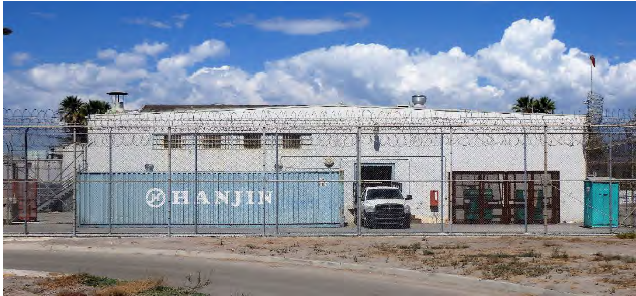
View of gymnasium, facing north.
