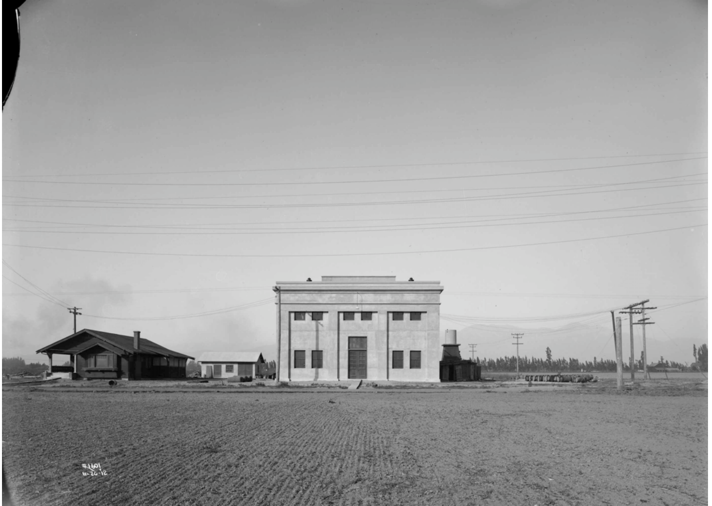
Historic photo of the Chino Substation – view north of the south (front) elevation, November 20, 1912. Image Source: Huntington Library Photo Archive – Southern California Edison Co. Collection (call #02-01601).
