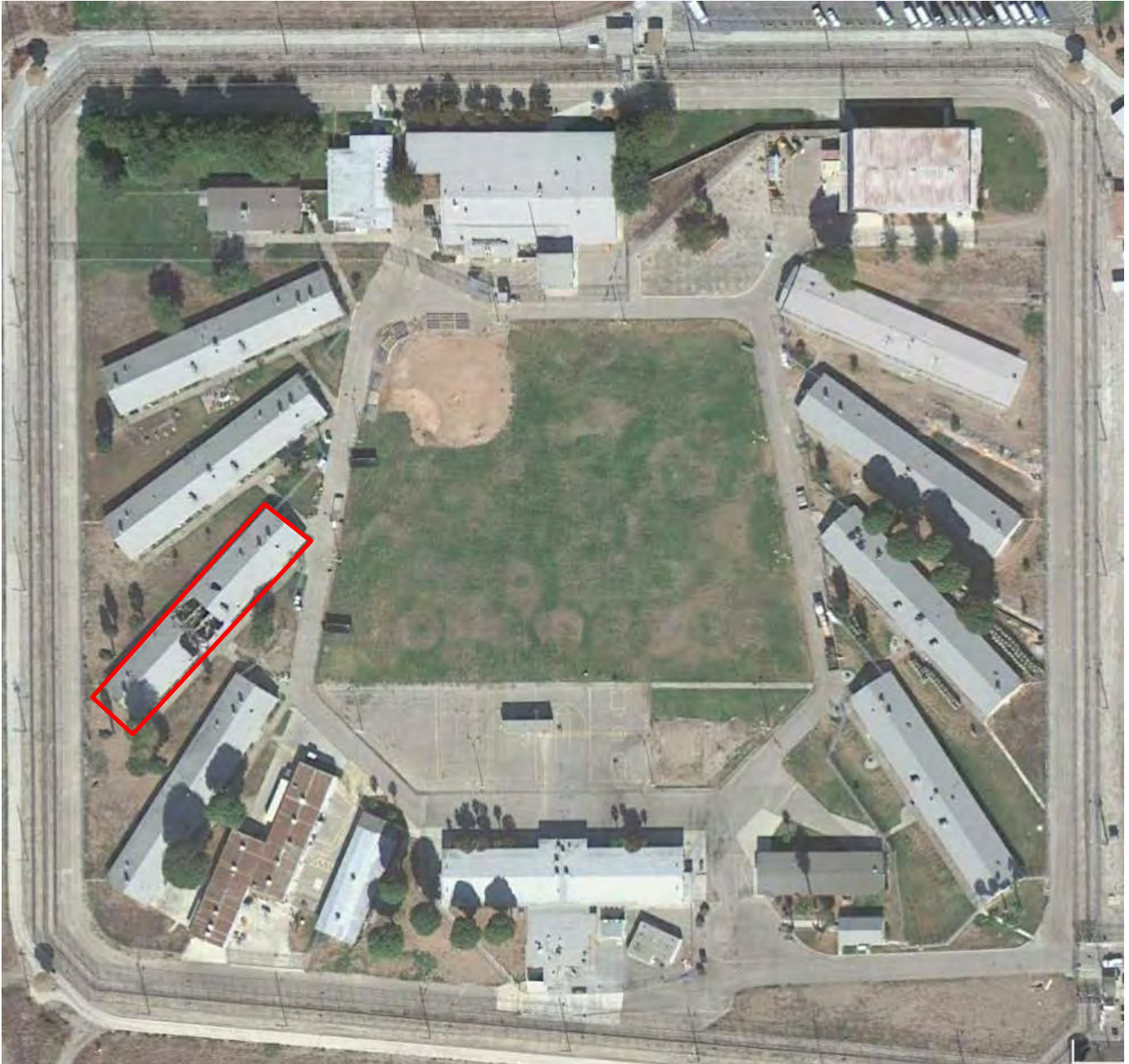
Facility A, November 2009. Damaged Joshua Dormitory in red.
