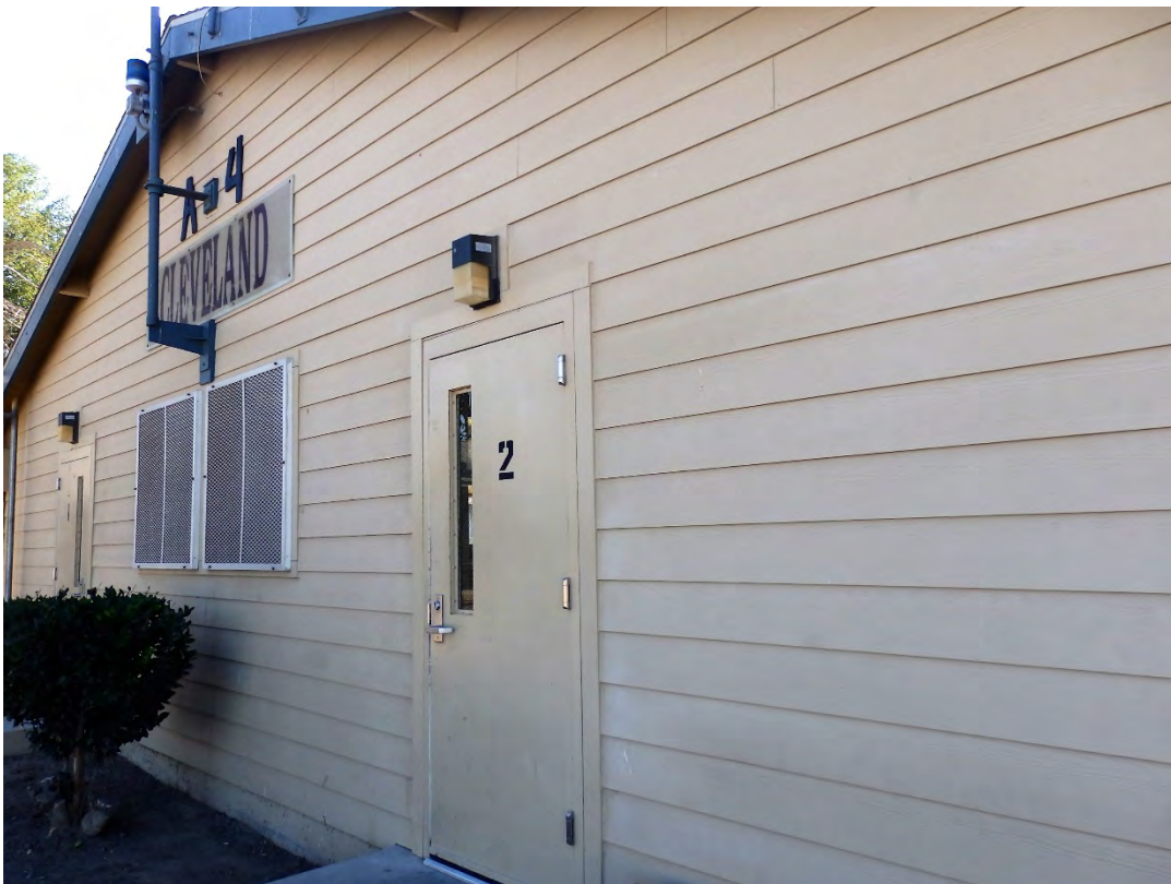
Building 388 Cleveland Dormitory
