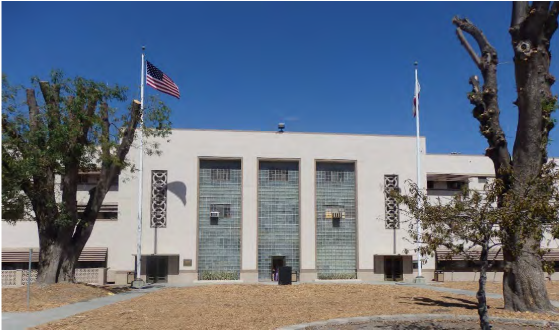
Central portion of administration building, showing glass brick walls.
