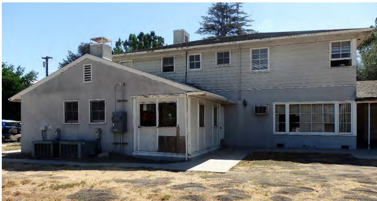
Rear of house, looking southeast at enclosed dining porch.
