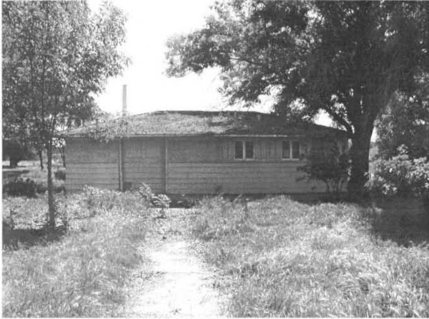
Figure #1) North (front) facade of Feature #1
