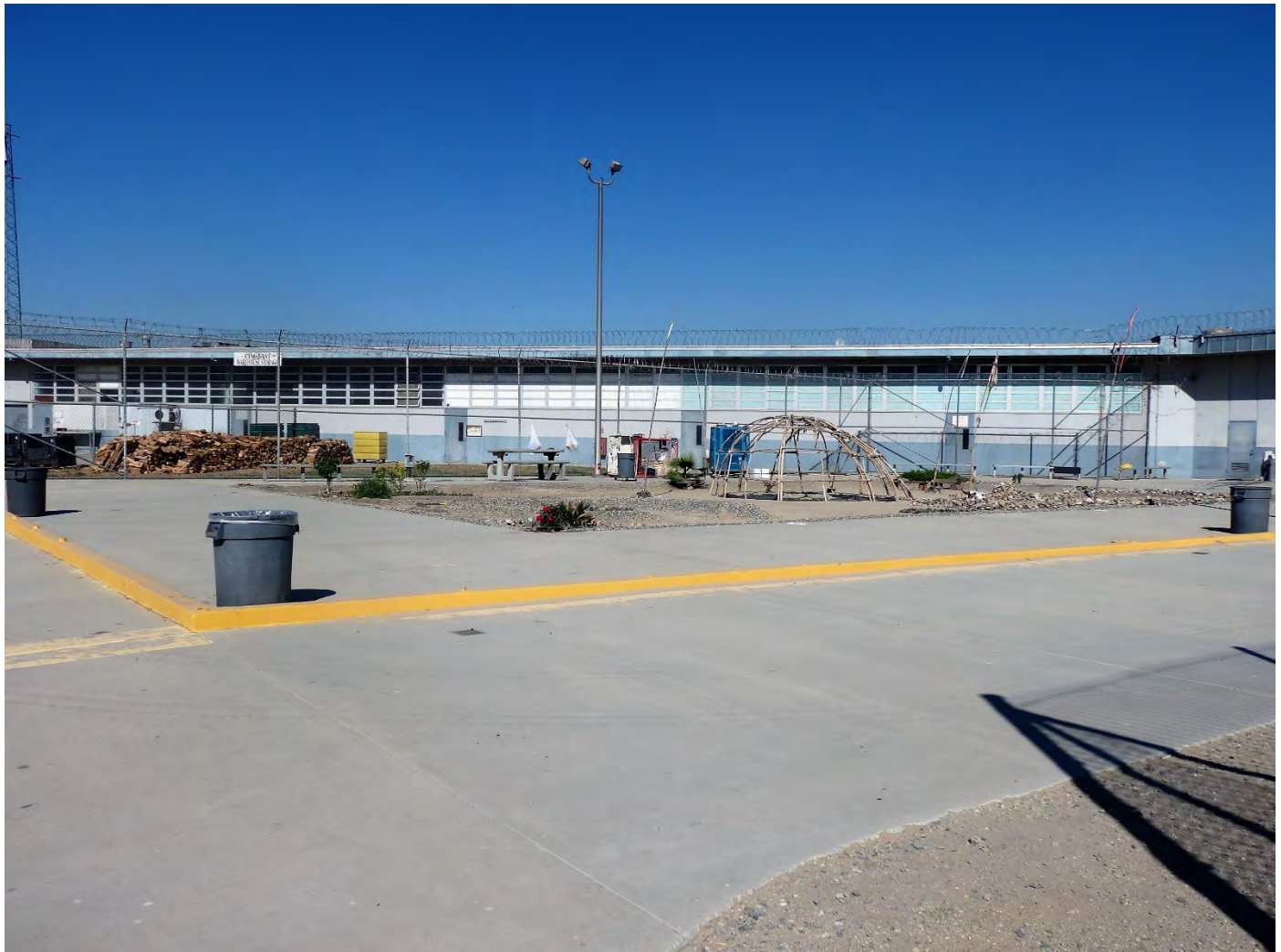
Old vocational maintenance and Prison Industry Authority area, western wing of Prison Industry Authority/education/gym/canteen building.
