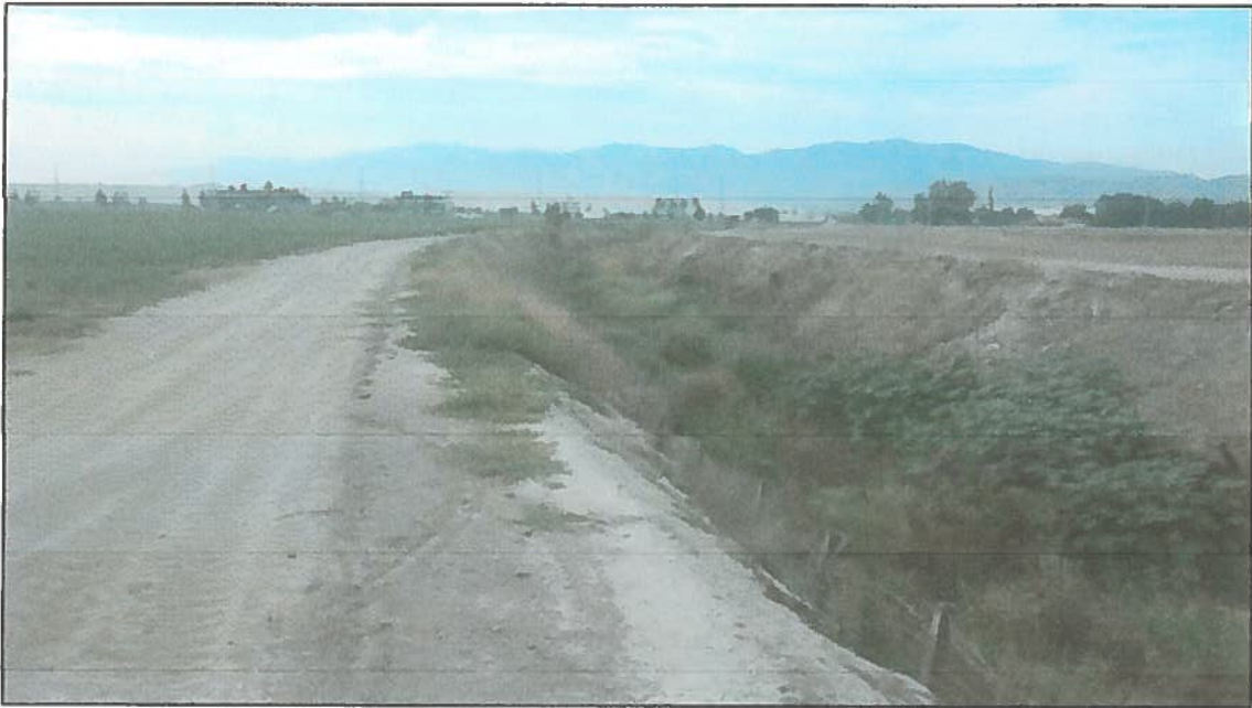
View south of the Cypress Channel north of Kimball showing the cut walls, railroad tie shoring and wire fence.
