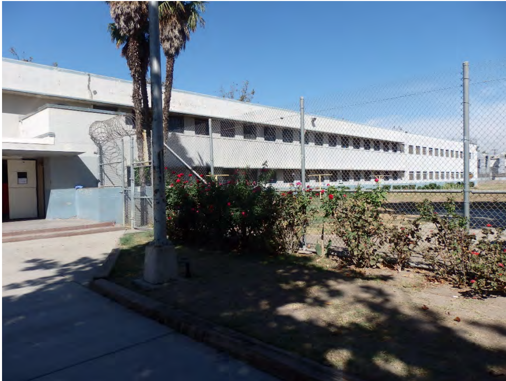
North end of building. Projecting cornice and balcony do not extend over northern-most 85 feet.
