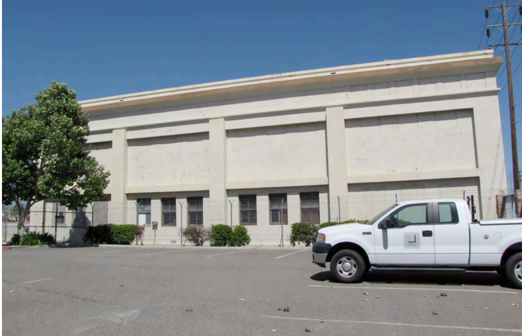
View east of the west elevation from the adjacent SCE parking lot where the Substation family homes were originally located. All second-story and frieze windows are painted over from the exterior. Some first-floor windows have been infilled, however, the fenestration dimensions are evident from cracking of the infill material.
