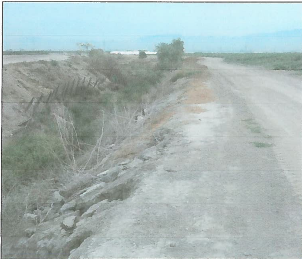
View north-northwest of the Cypress Channel showing the cut walls, railroad tie shoring and wire fence.
