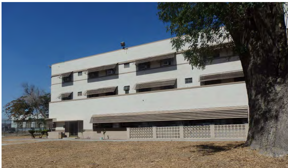
West end of administration building.
