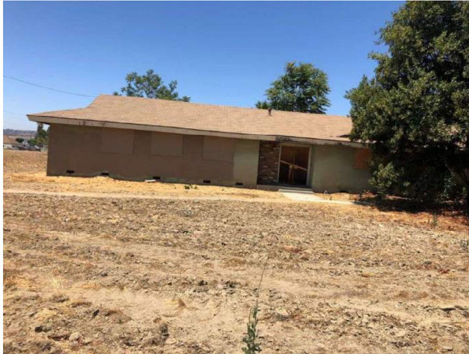
Photograph 1: View looking west at the front elevation of the residence from East End Avenue.
