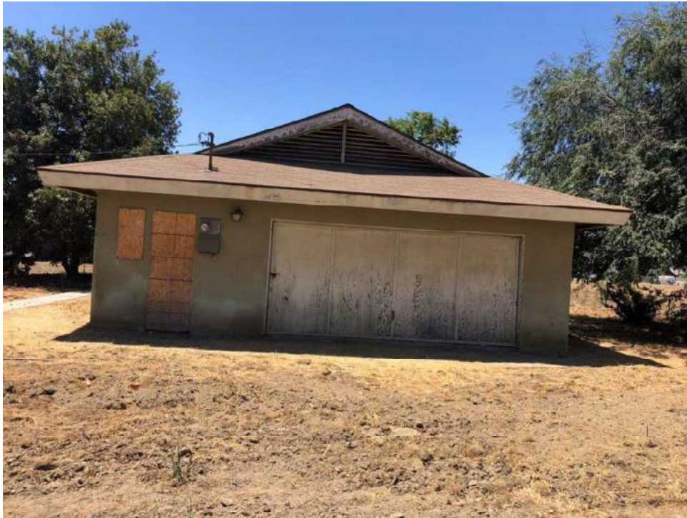
Photograph 3: View looking west at the attached two-car garage.
