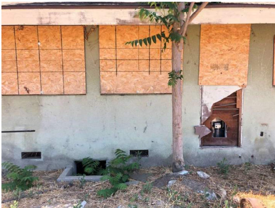
Photograph 6: View looking at wall surfaces and boarded windows.
