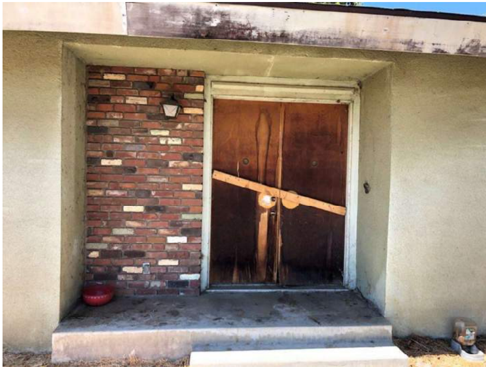
Photograph 5: Close-up of the front entry on the building's east elevation facing East End Avenue.
