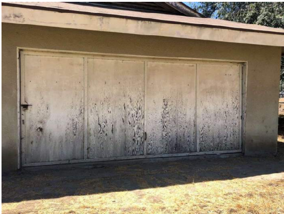
Photograph 8: Close-up of the east elevation garage door.
