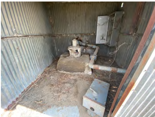
17. Well shed interior
