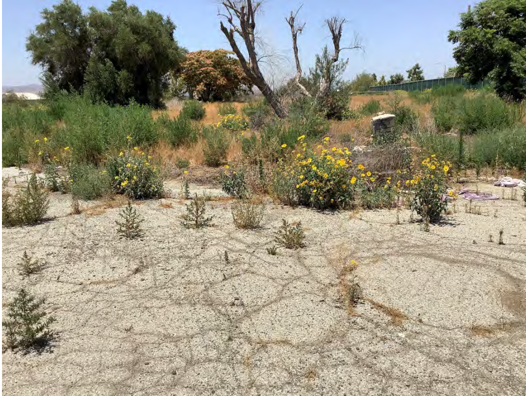
Figure 6-10. Portion of asphalt driveway south of Remington Avenue, facing west.
