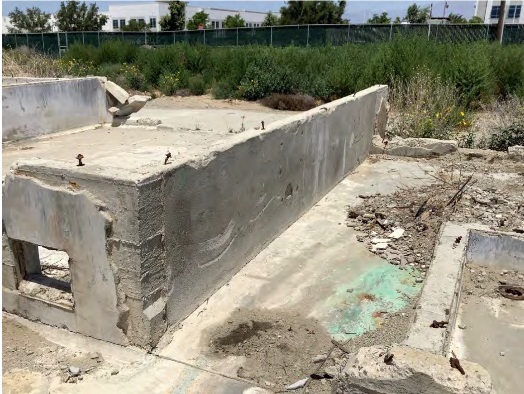
Figure 6-7. Eastern portion of milking barn (Feature 1), facing north.
