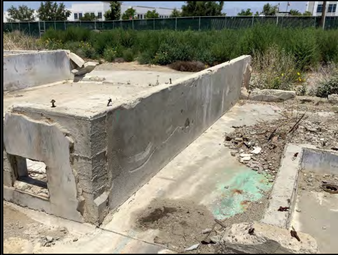
Eastern portion of milking barn (Feature 1), facing north.
