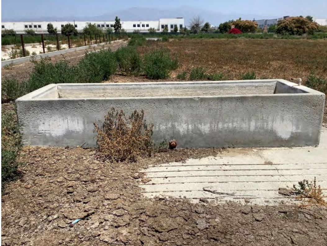
Figure 6-12. Concrete water tank adjacent to western feed driveway (Feature 5), facing north.
