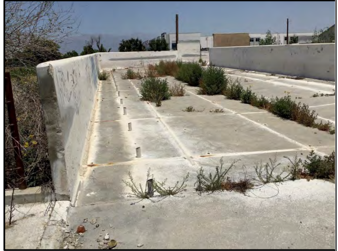
Feature 2, holding pen adjacent to milking barn, facing north.
